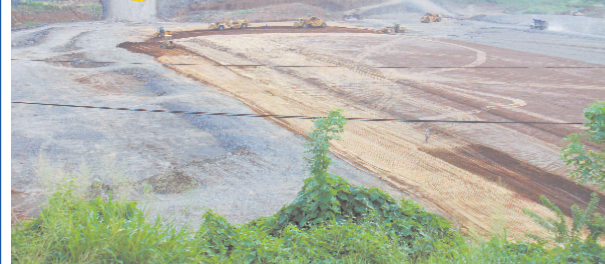
THE RUNWAY begins to take shape in the 1st kilometer.
