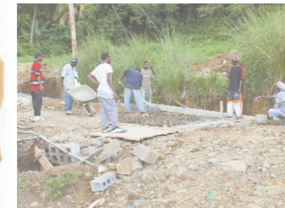
WORKERS with the HLDC installing drains at Carapan.
