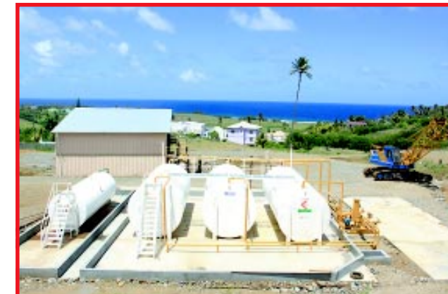
The new fuel station located on the project site
