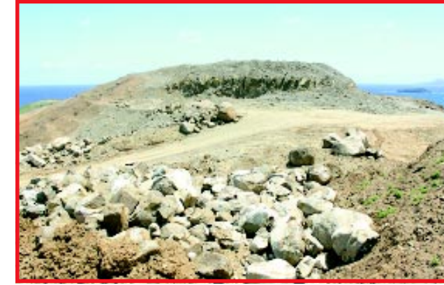
The Hills come down as excavation work continues
