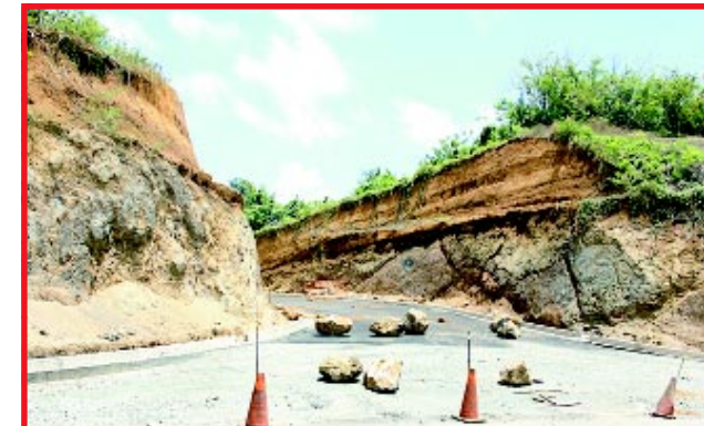
Work in progress on the New Windward Highway
