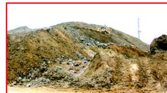
Excavation being done in the Mt. Coke area
