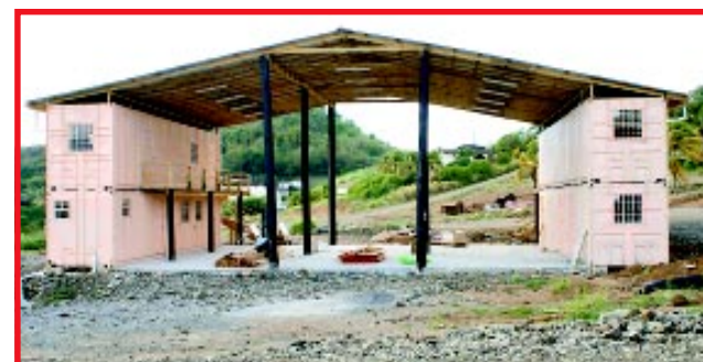
The Workshop located on the project site
