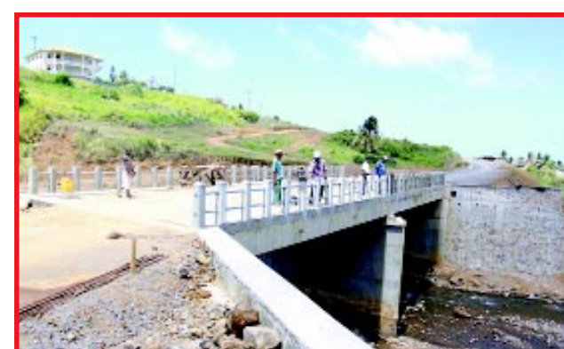
The new Argyle Bridge on the Windward Highway
