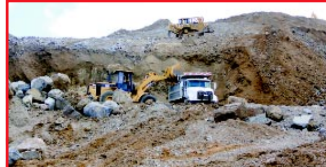
More, excavation work
