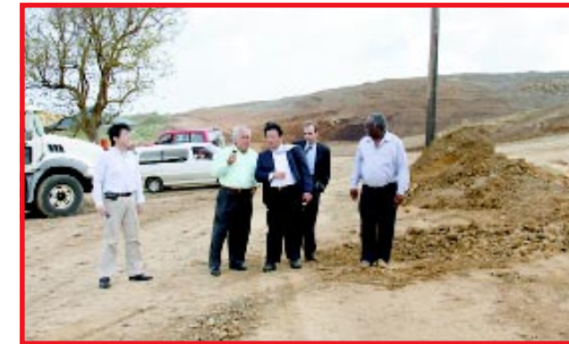
Engineers from Taiwan's Engineer and Consulting company CECI, on a recent visit to the project site
