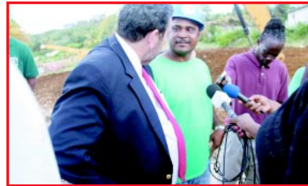
P.M. Gonsalves, meets Vincentian Konrad Sam, said to be the best heavy equipment operator on the project
