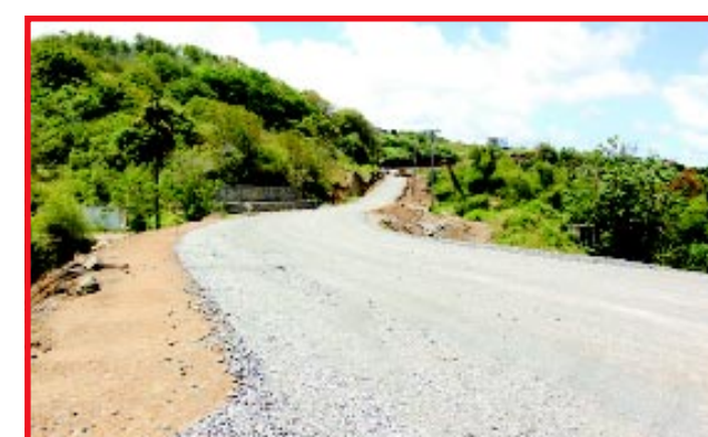
The New Windward Highway, nearing completion
