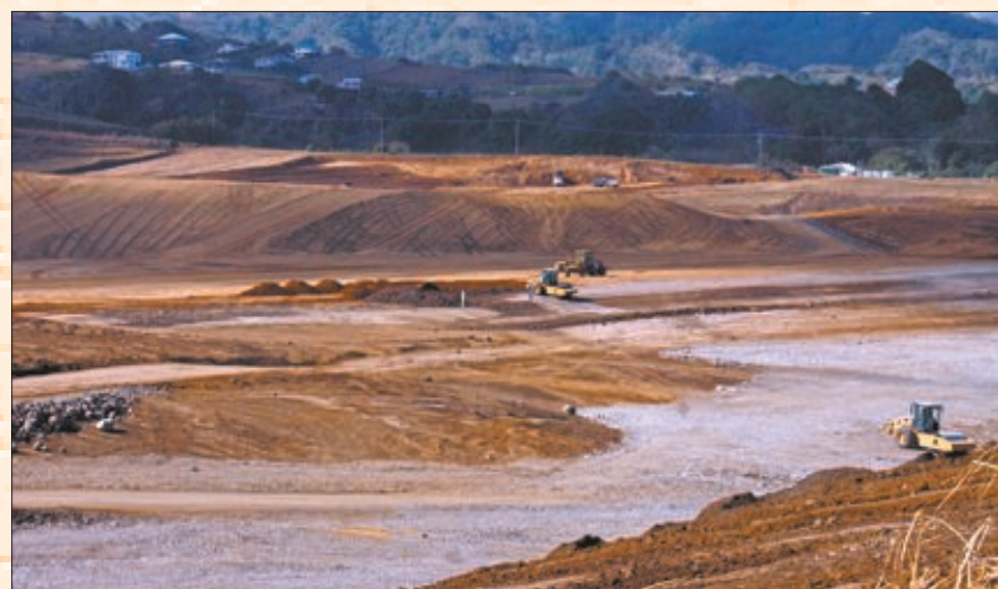
Top soil being removed in the 2nd kilometer as the area is prepared for the construction of the terminal building
