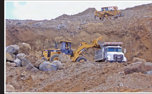
MORE ROCKS being removed from McConnie Yammie Hill.
