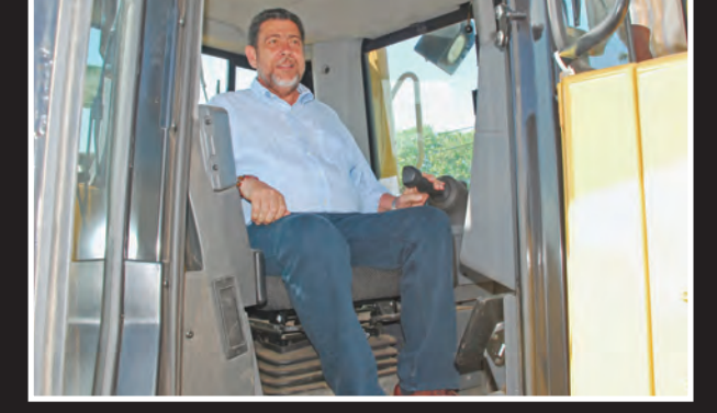
PRIME MINISTER Dr. Ralph Gonsalves seated in a bulldozer as he prepares to demolish a building.
