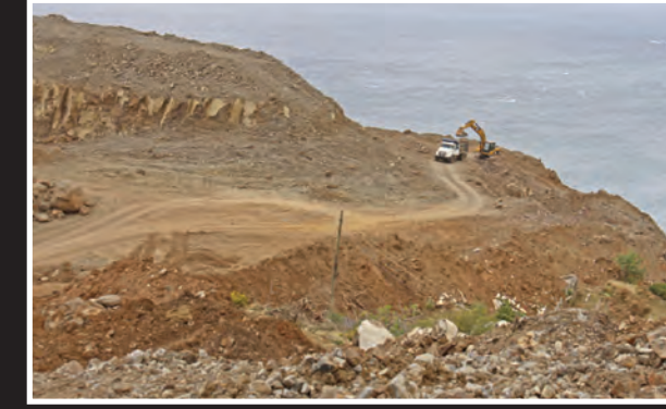
EARTHWORKS being carried out on Fort Hill.
