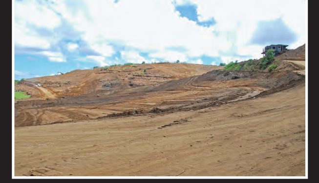
EARLY STAGES of earthworks in the 1st kilometer.
