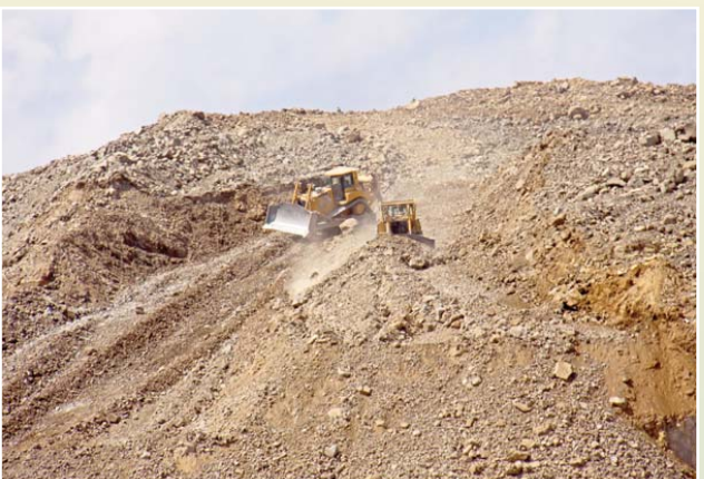
Pushing the fractured rocks off Fort Hill.
