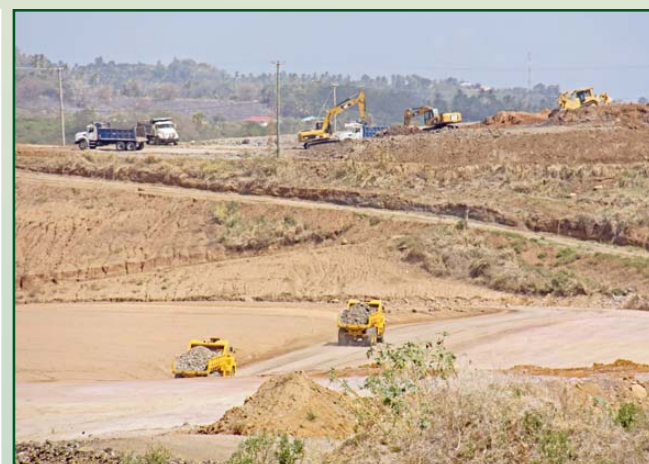
Working on Johnson Hill/Rocks en route to the 2nd kilometer.
