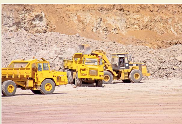
Loading the rocks onto trucks for transport to the 2nd kilometer.
