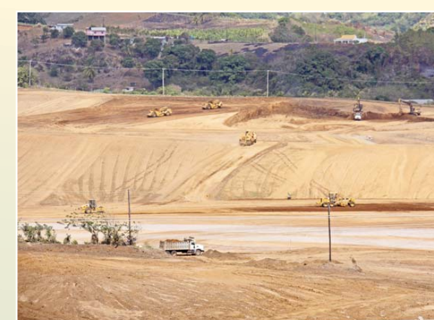
Removal of top soil in the 2nd kilometer.
