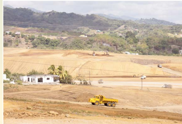
Work continues apace in the 2nd kilometer.
