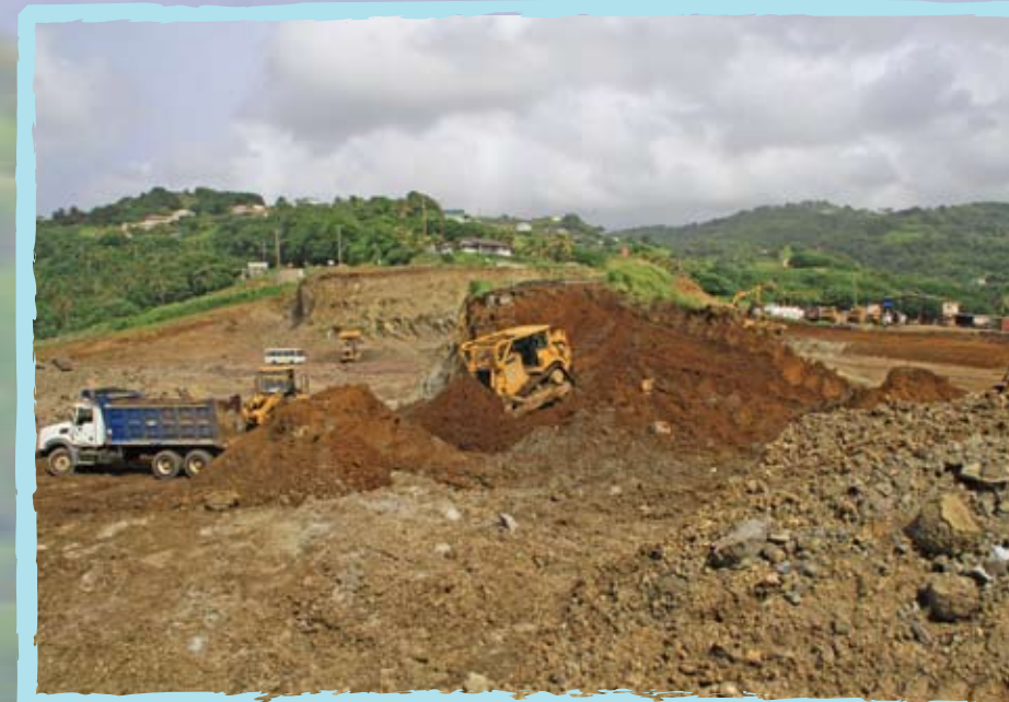
Excavating the area around the old Windward Highway
