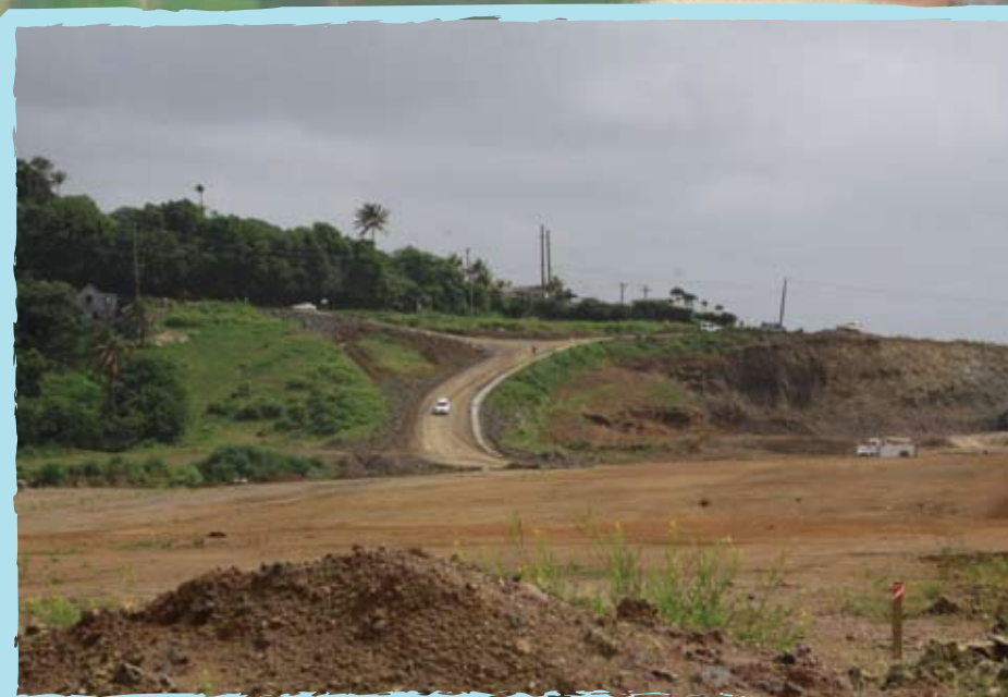
Entrance to the new bypass road
