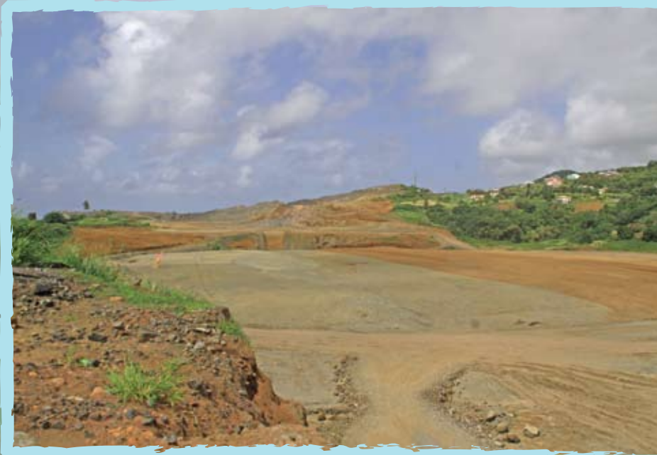
The 1st kilometer of the project
