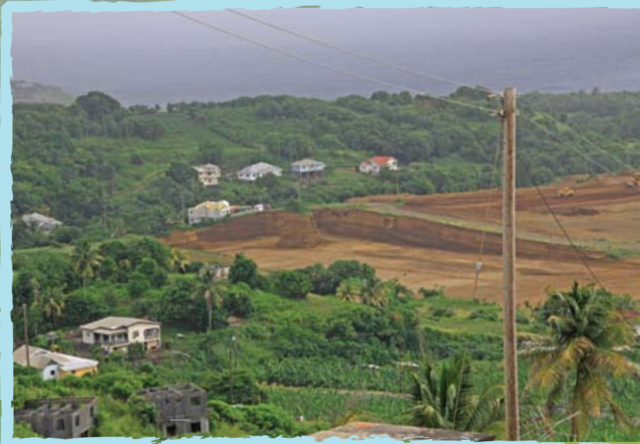
Overlooking the area earmarked for construction of the terminal building
