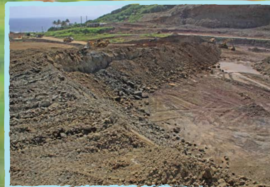
Removing the old Windward Highway
