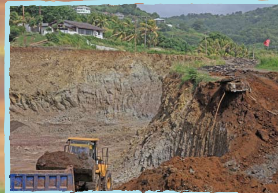
Breaking the old Windward Highway
