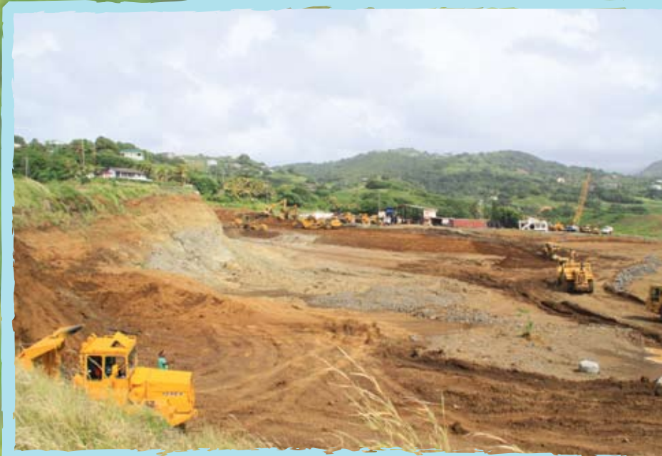
Excavating below the old Windward Highway prior to its removal
